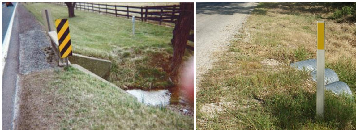
Figure 7-6 Sample Culvert End Marker Signs
