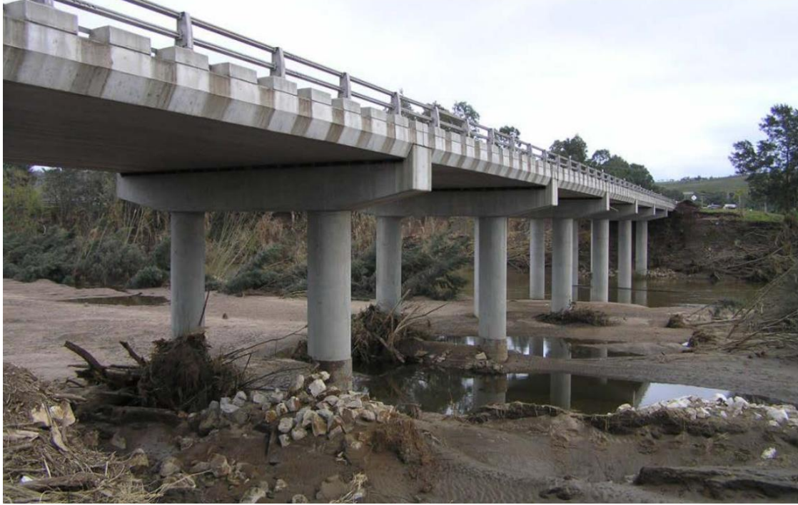
Plate 13.16 Excessive scour due to significant constriction of waterway
