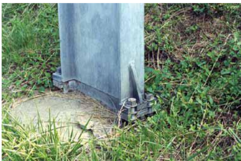
Plate 12.53 Typical unidirectional slip base
