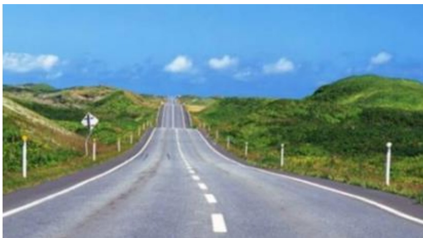
Plate 5.27 Poor alignment showing optical breaks caused by steep sag curves and horizontal tangent
