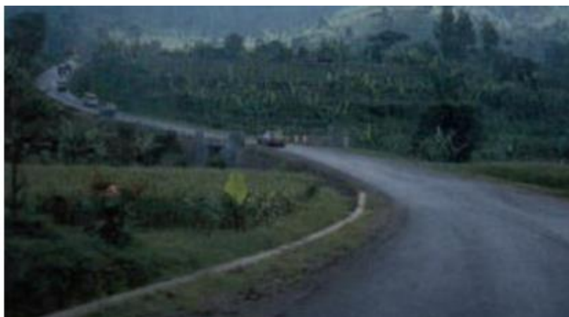
Plate 5.28 Example of good combination of horizontal and vertical curve
