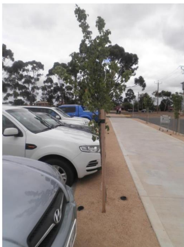
Plate 11.6 Narrow landscaping area does not allow for vehicle overhang
