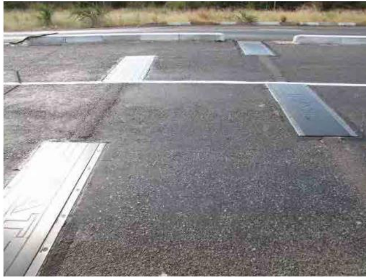
Plate 11.15 Typical High Speed WIM Device (Bending Plate)
