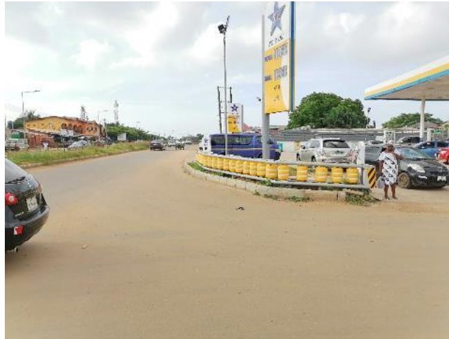
Plate 12.14 Mountable kerbs in front of roller barrier
