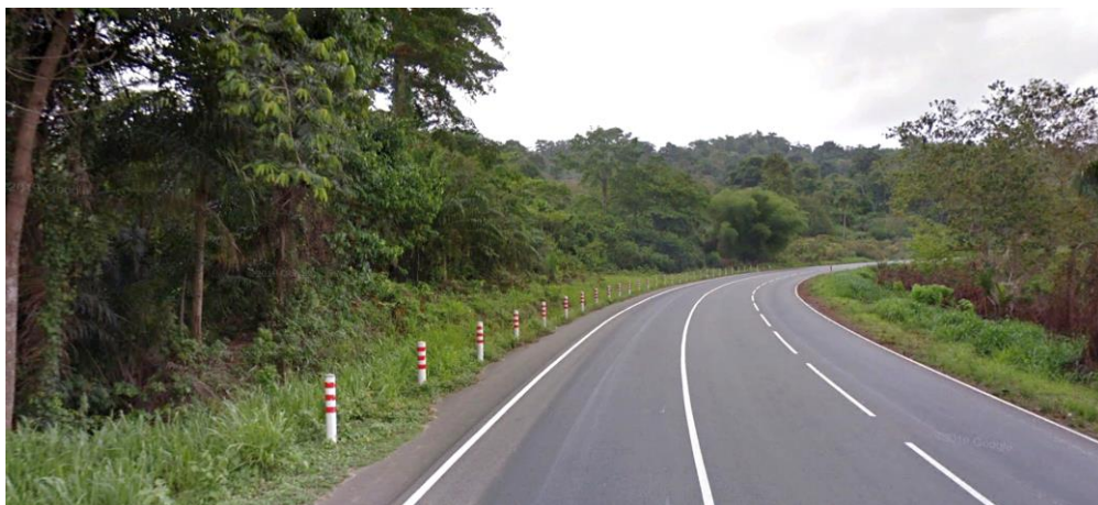
Plate 5.35 The use of Bollards as safety fence is inappropriate for traffic safety
