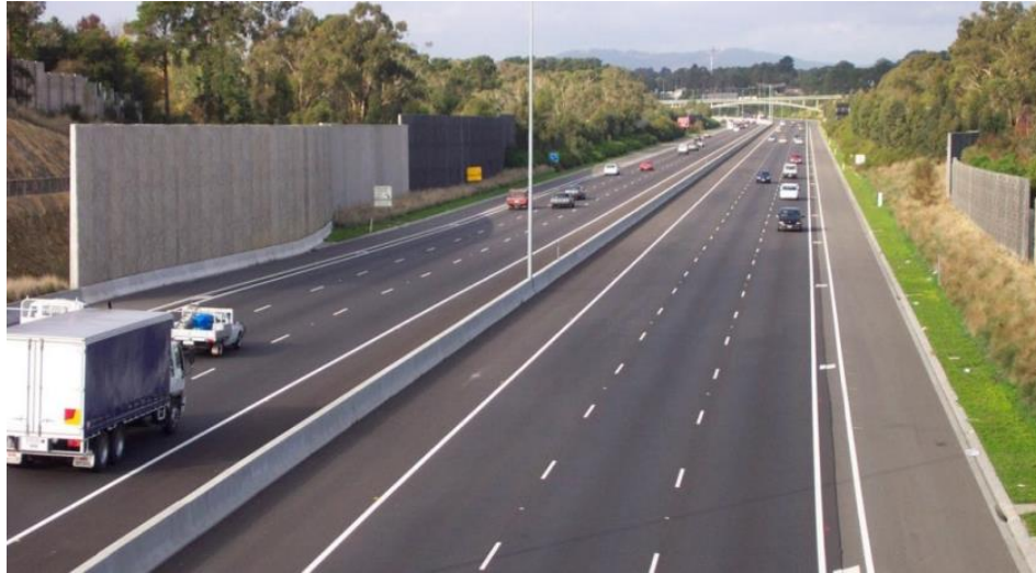
Plate 12.45 Textured and coloured concrete noise walls on an urban expressway/motorway
