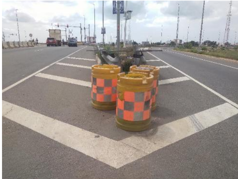
Plate 12.39 Sand filled plastic barrel attenuators located at a gore
