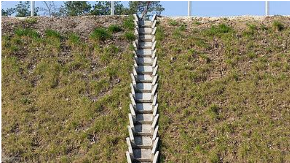
Plate 13.6 Batter drain
