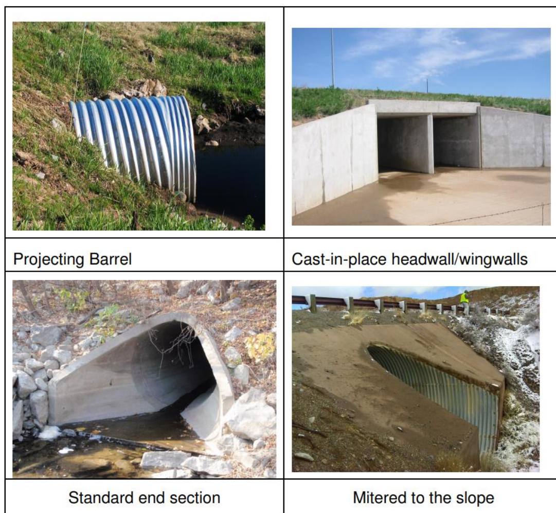
Plate 13.11 Four standard inlet types
