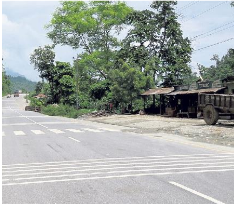
Plate 10.5 Jiggle bars in thermoplastic/line flex
