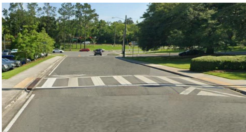
Plate 10.2 Trapezoidal Road hump with drainage slot at both ends
