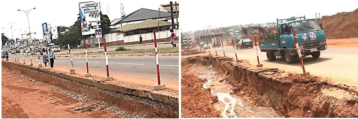
Plate 5.6 Absence of lateral buffer along active work zones
