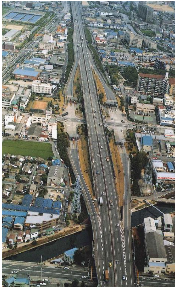
Plate 9.3 Typical Four -Leg Diamond Interchange (Amagasaki, Japan)
