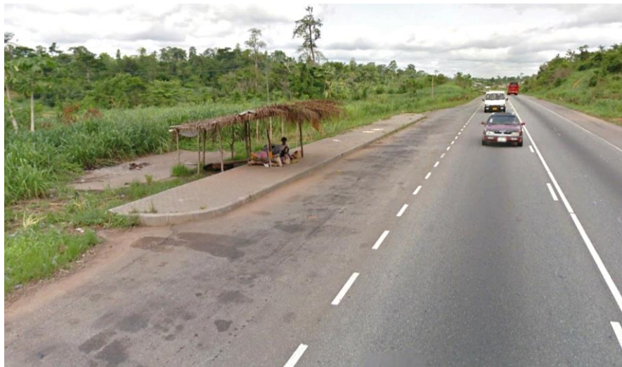
Plate 5.20 Rural bus bay provides safe off-road operation
