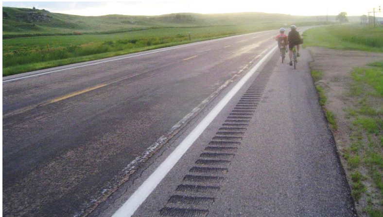
Plate 5.25 Paved shoulder with rumble strips
