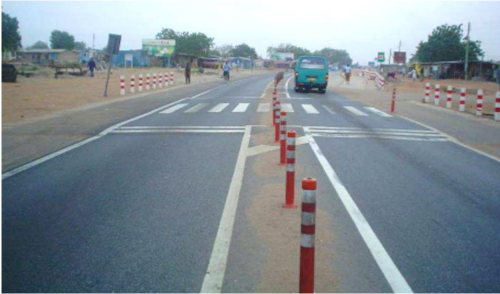
Plate 10.3 Pedestrian crossing placed on top a trapezoidal hump
