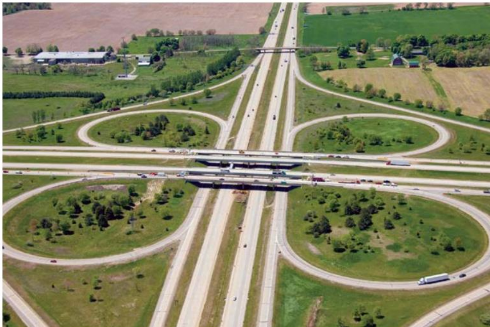
Plate 9.12 Four-Leg Interchange, Cloverleaf with Collector–Distributor Roads
