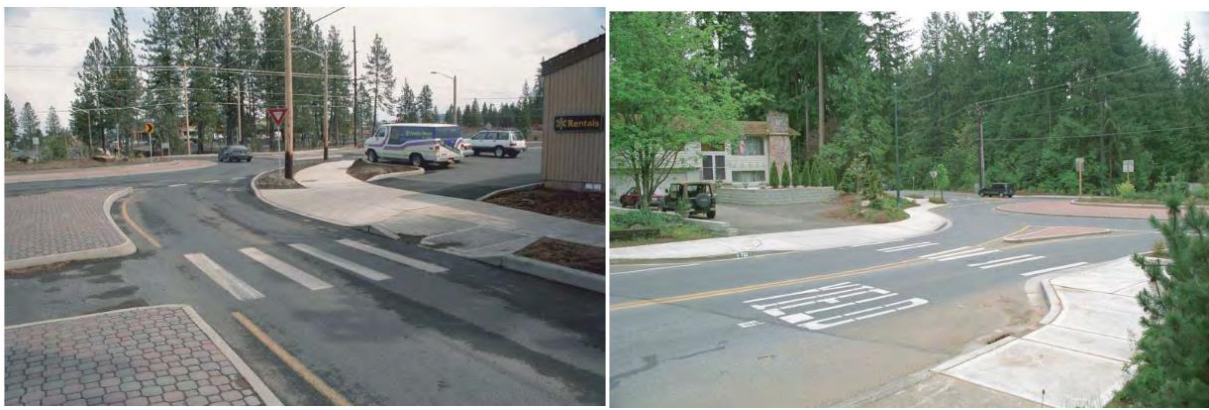
(a) Access between crosswalk and roundabout
