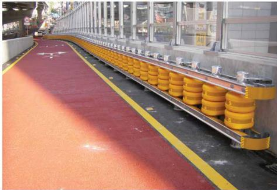
Plate 12.11 Wall mounted roller barriers
