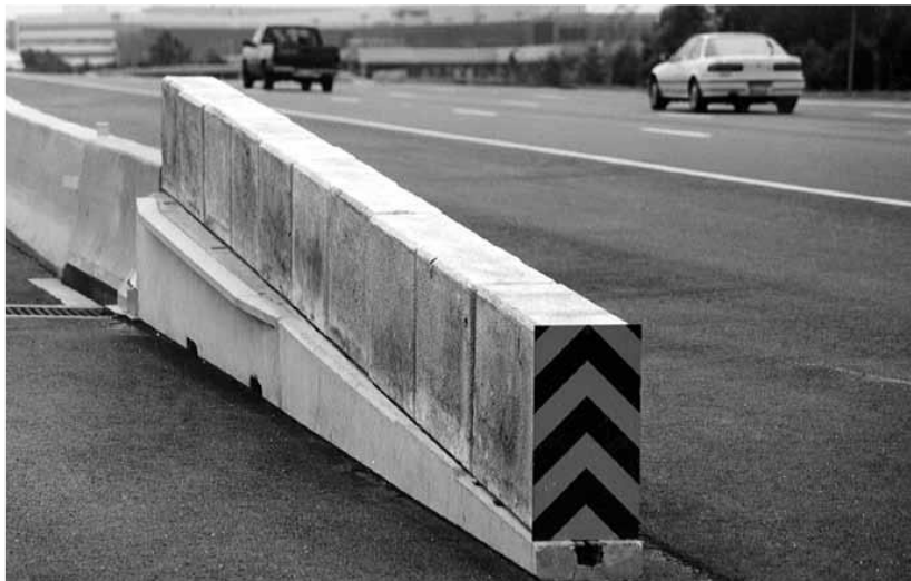
Plate 12.29 Advanced Dynamic Impact Extension Module (ADIEM™)
