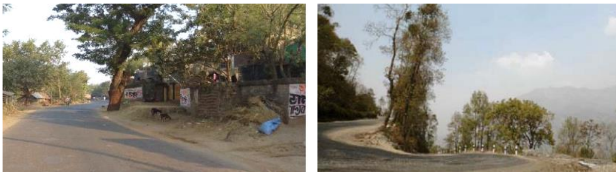
Plate 5.26 Tree located too close to the carriageway on inside of curve
