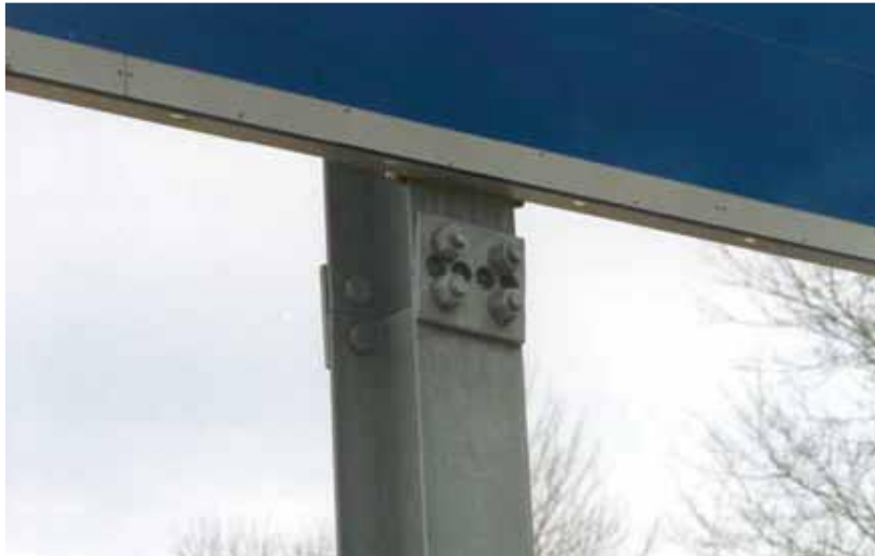
Plate 12.55 Perforated fuse plate design
