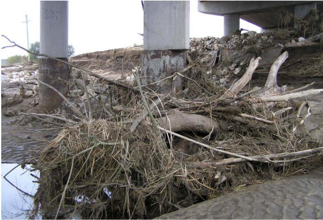
Plate 13.18 Example of local scour at piers
