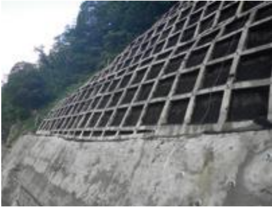
Plate 11.23 Grating Crib Works and Rock Bolt Works
