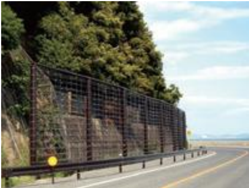
Plate 11.24 Rockfall Protection Fence
