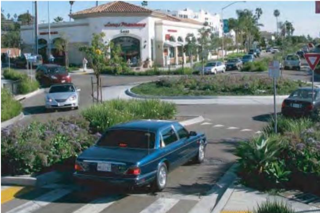
Plate 8.24 Example of Splitter Island Landscaping Encroaching on Sight Lines
