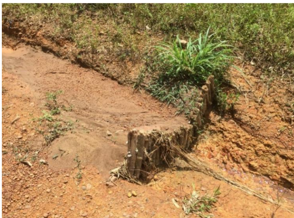
Plate 13.10 Scour check made from wooden stakes
