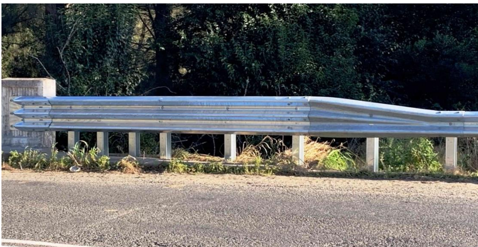
Plate 12.27 Transition between W-Beam safety barrier and concrete parapet
