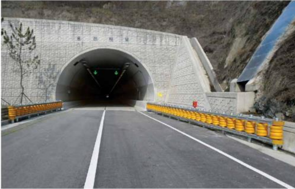
Plate 12.13 Roller barrier installed at the approach to a tunnel
