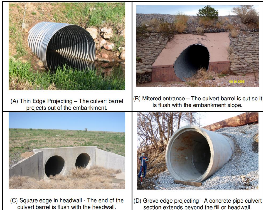
Plate 13.12 Typical inlet configurations.
