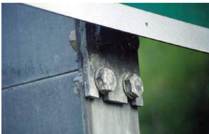
Plate 12.54 Slotted fuse plate design
