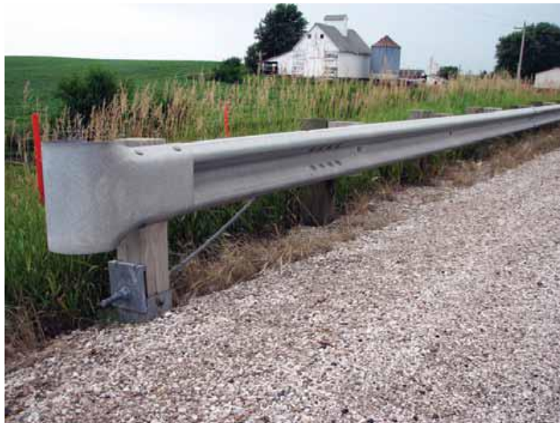
Plate 12.15 Training end w-beam guardrail anchorage
