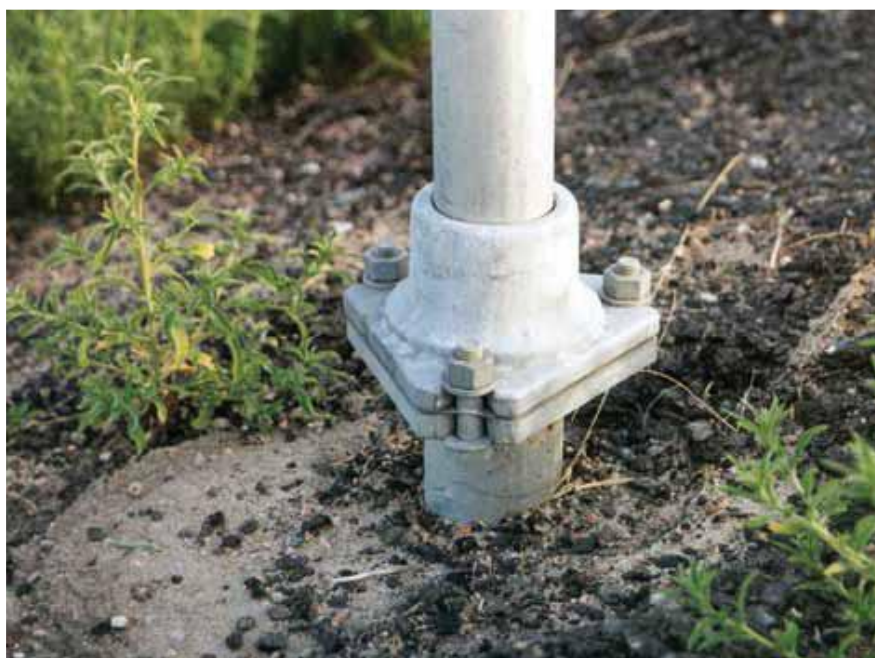
Plate 12.57 Multidirectional Slip Base for Small Signs
