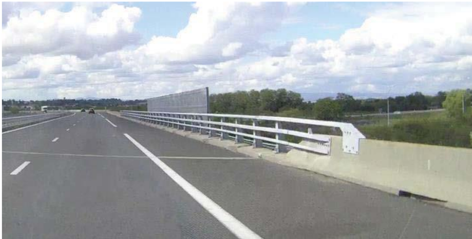
Plate 12.26 Transition between concrete safety barrier and metal parapet
