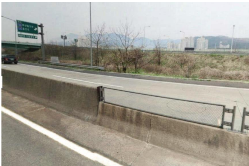
Plate 12.51 127mm high concrete Safety barrier as Anti-Glare System
