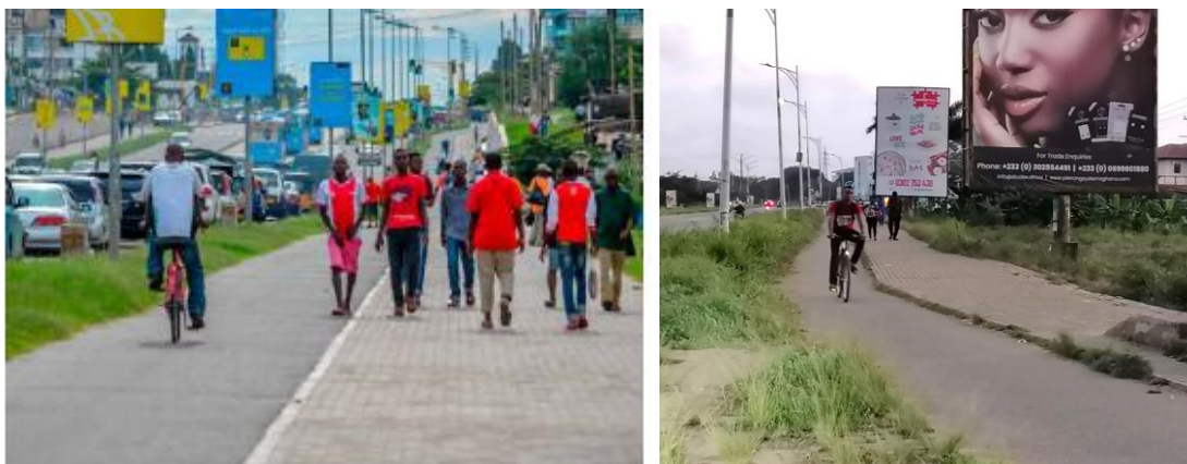
Plate 5.8 Separation and protection of both pedestrians and cyclists from high-speed road
