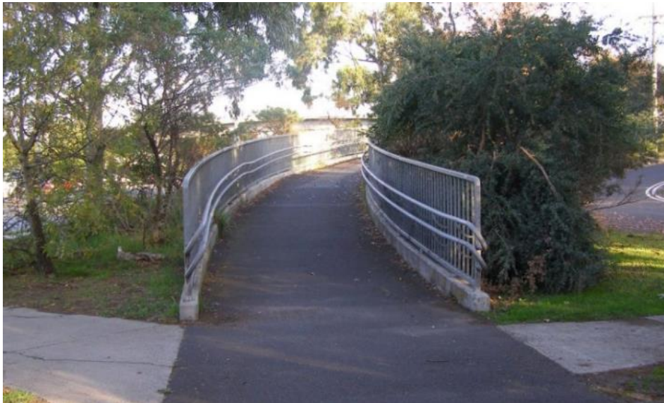
Plate 12.44 Rails and kerbs to cater for impaired people on a ramp to an overpass
