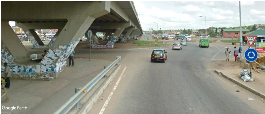
Plate 5.52 Unsafe roundabout with no deflection on the approach splitter island
