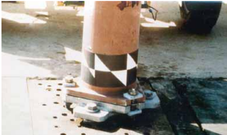
Plate 12.60. Example of a Luminaire Slip Base Design
