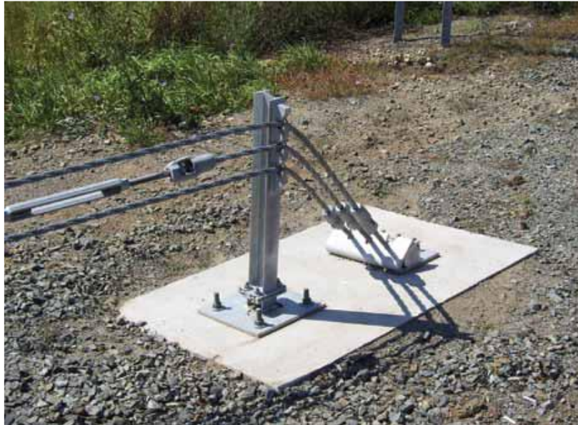
Plate 12.16 Terminals for high tension cable barrier systems
