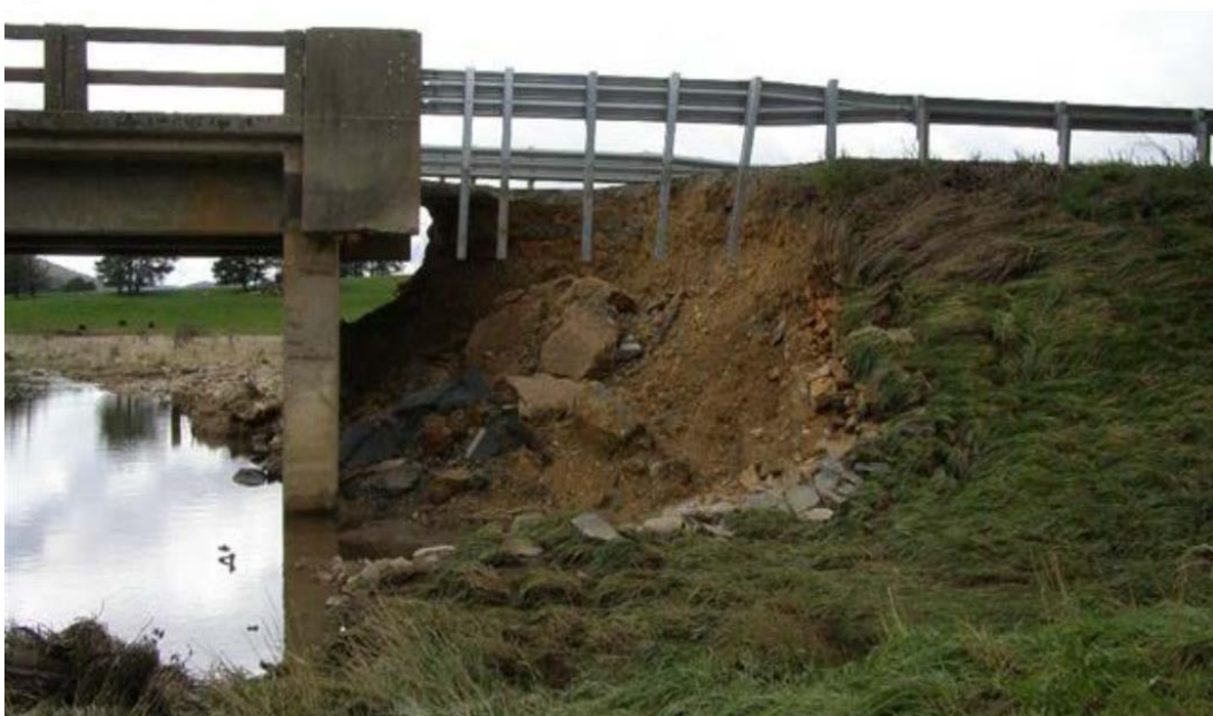
Plate 13.19 Example of local scour at an abutment
