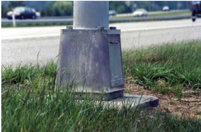
Plate 12.59. Example of a Cast Aluminium Frangible Luminaire
