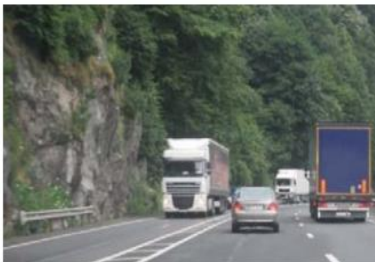
Plate 5.33 Highway with painted median
