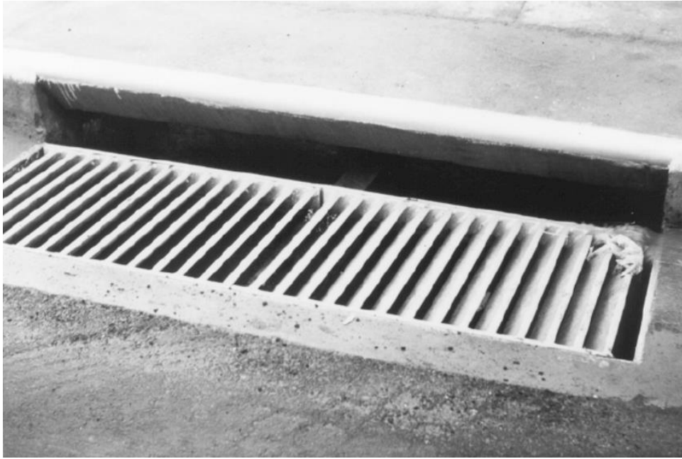
Plate 13.3 Combination kerb-opening, 45 degree tilt-bar grate Inlet.
