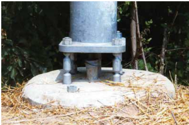
Plate 12.61 Example of a Frangible Coupling Design
