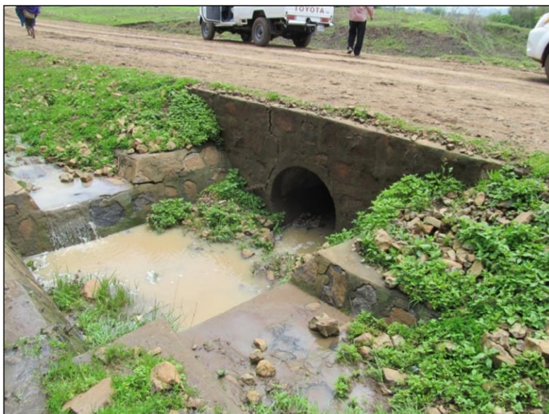
Plate 13.9 Catch pit inlet structure
