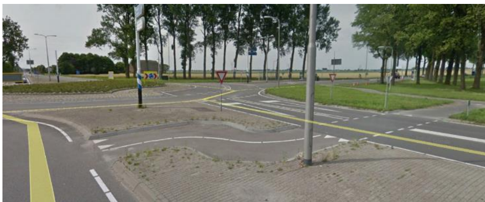
Plate 8.21 Example of a chicane in a splitter island at a turbo roundabout in the Netherlands
