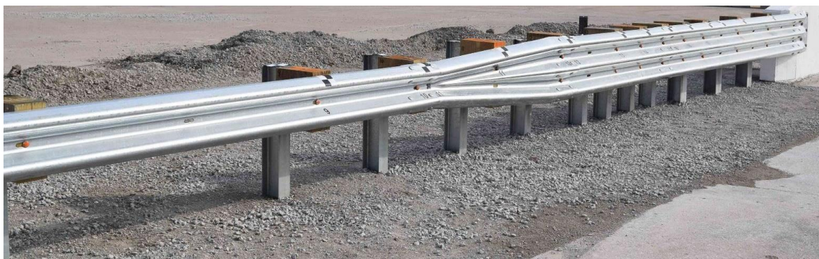
Plate 5.38 Safe connection between guardrail and rigid barrier on bridge
