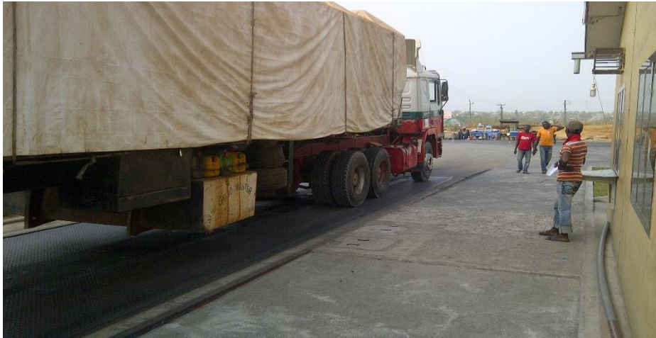
Plate 11.8 Typical 3.2 m × 22 m Multi-deck Weighbridge
