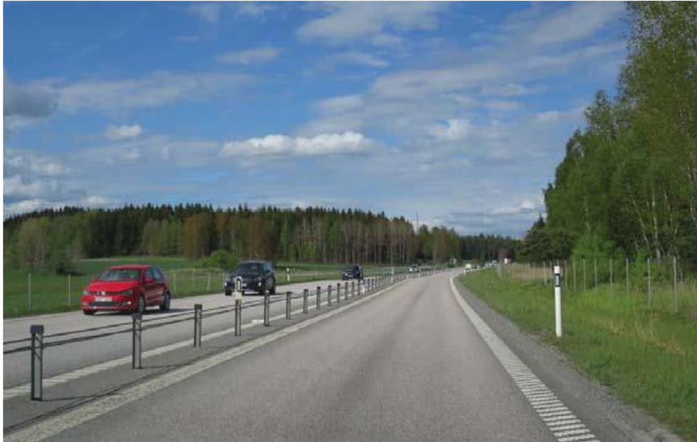
Plate 7.2 “2+1” Road with median safety barrier
