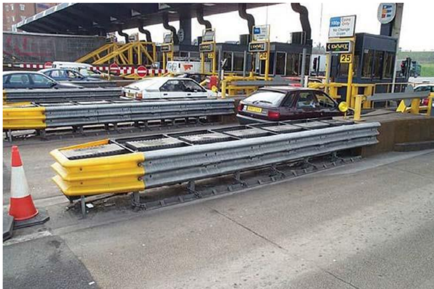
Plate 11.20 Impact attenuator installed at approach of toll island
