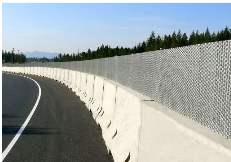
Plate 12.49 Safety Barrier mounted Anti-Glare Nets
