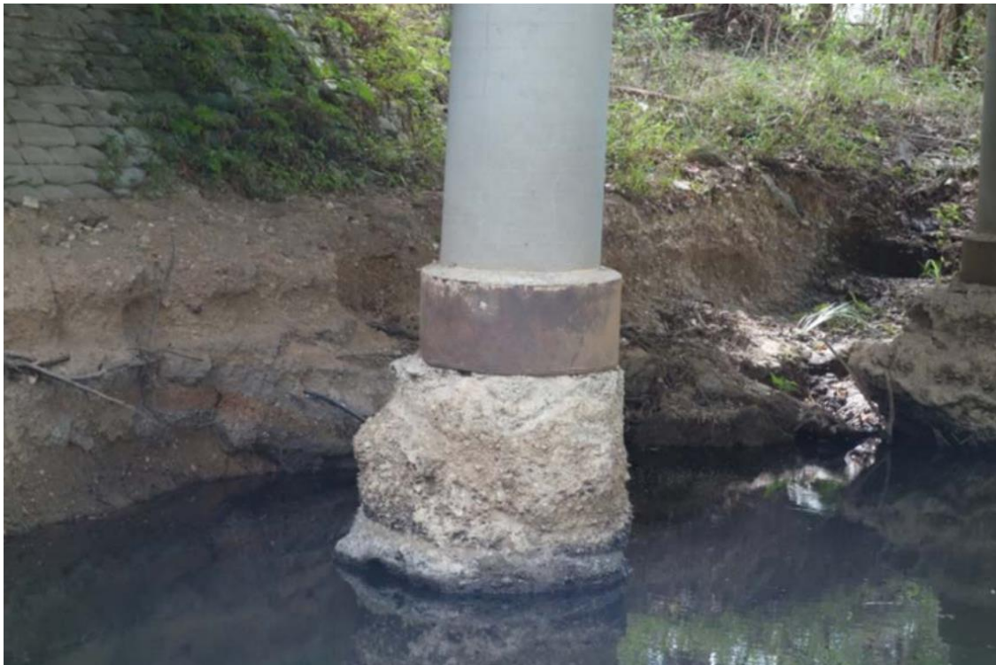
Plate 13.17 Local scour at a bridge pier due to significant constriction of waterway
