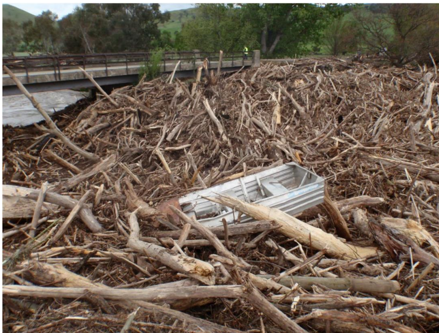
Plate 13.14 Debris accumulated upstream of a bridge
