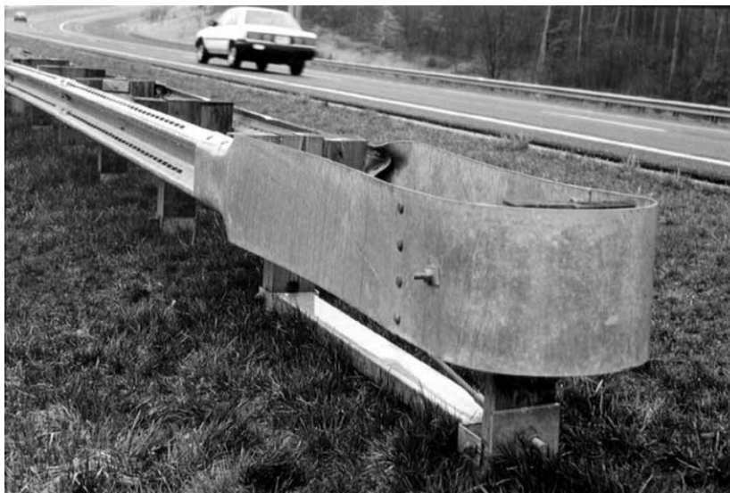
Plate 12.22 Crash Cushion Attenuating Terminal (CAT-350™)
