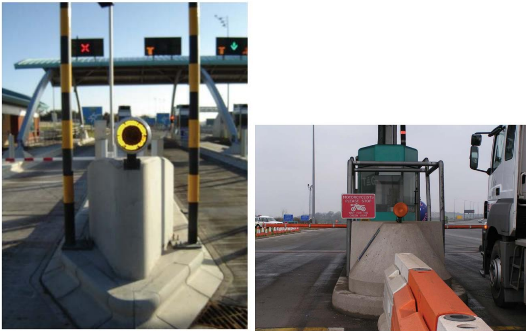
Plate 11.18 Hazard Warning Beacons Fixed to Concrete Bollard
