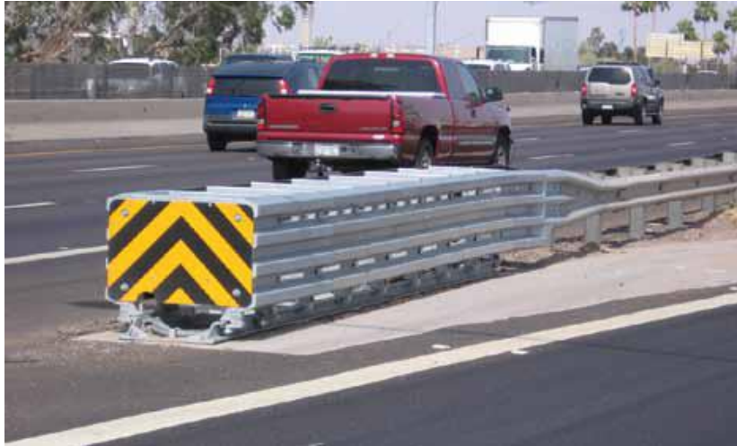
Plate 12.37 Smart Cushion Innovations (SCI-100GM) Crash Cushion
