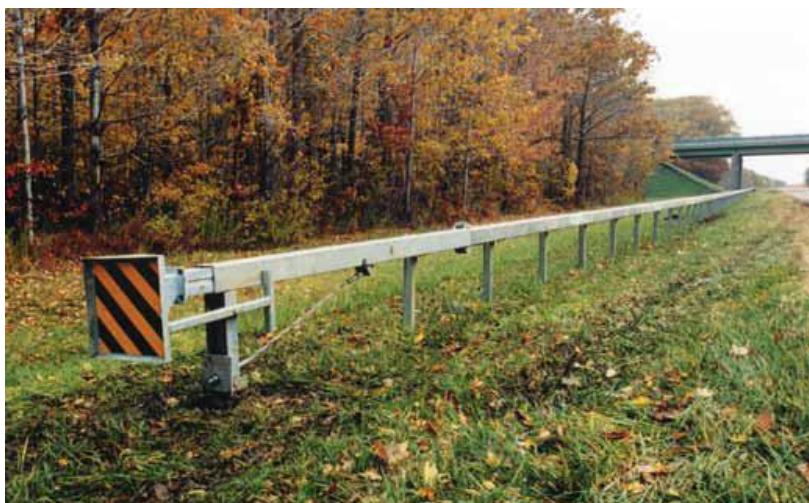
Plate 12.20 Bursting energy absorbing terminal
