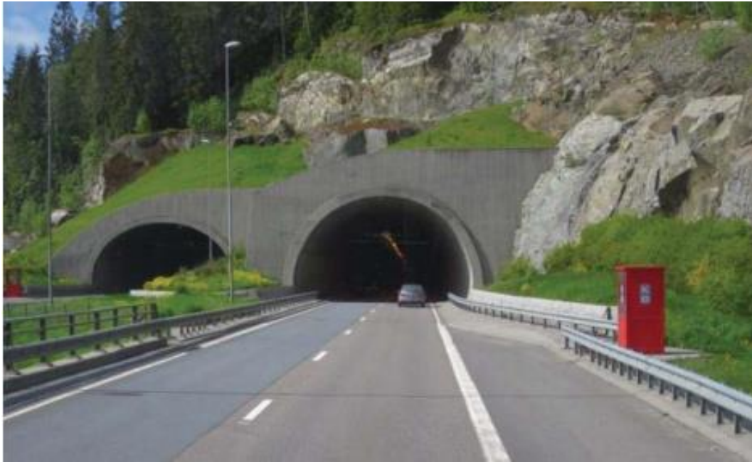
Plate 6.7 Double safety barriers and access opening at tunnel entrance
