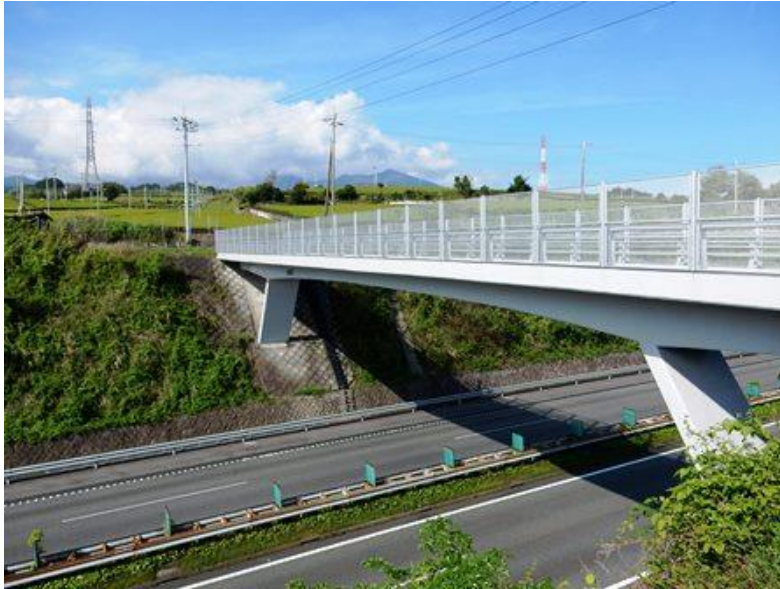
Plate 9.1 Typical Grade Separation with Open-End Span (Tomei Expressway, Japan)
