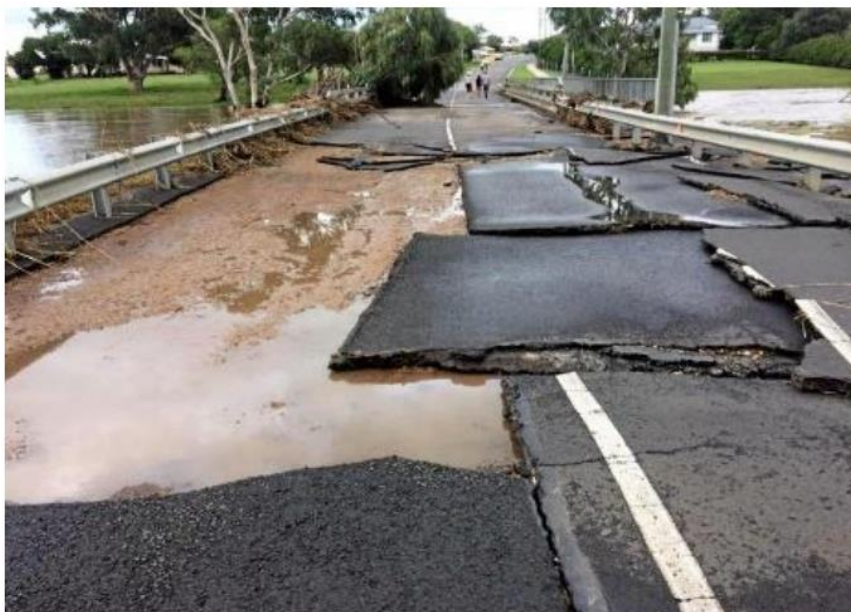
Plate 13.23 Example of floodway crossing damage starting from the upstream side of the floodway crossing
