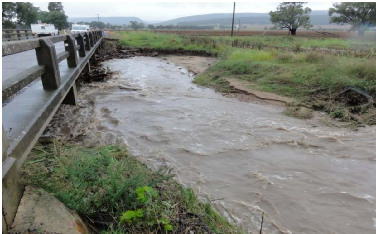
Plate 13.15 Scour at a highly skewed bridge
