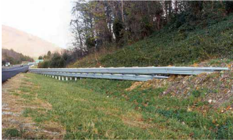
Plate 12.18 W Beam guardrail anchored in back slope
