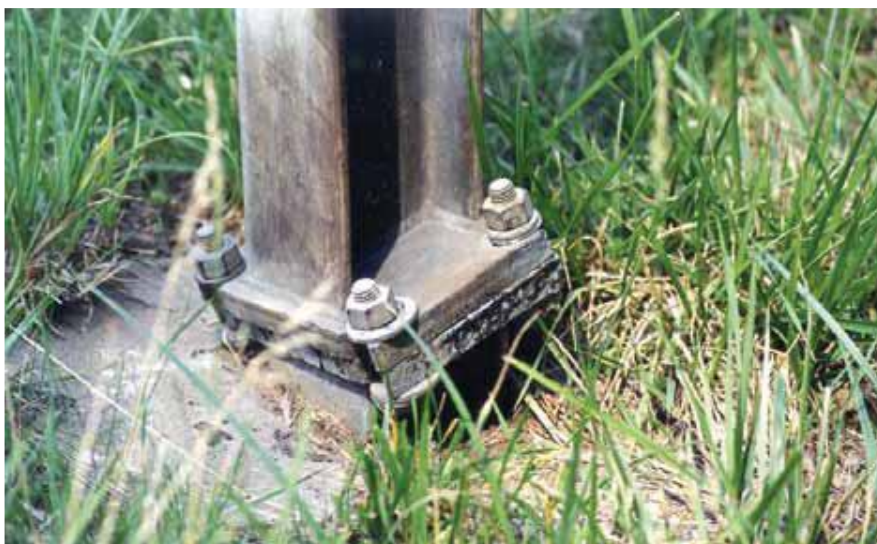
Plate 12.56 Unidirectional Slip Base for Small Signs
