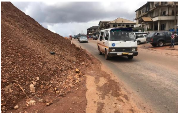
Plate 5.7 The material on the road is inappropriate for traffic safety
