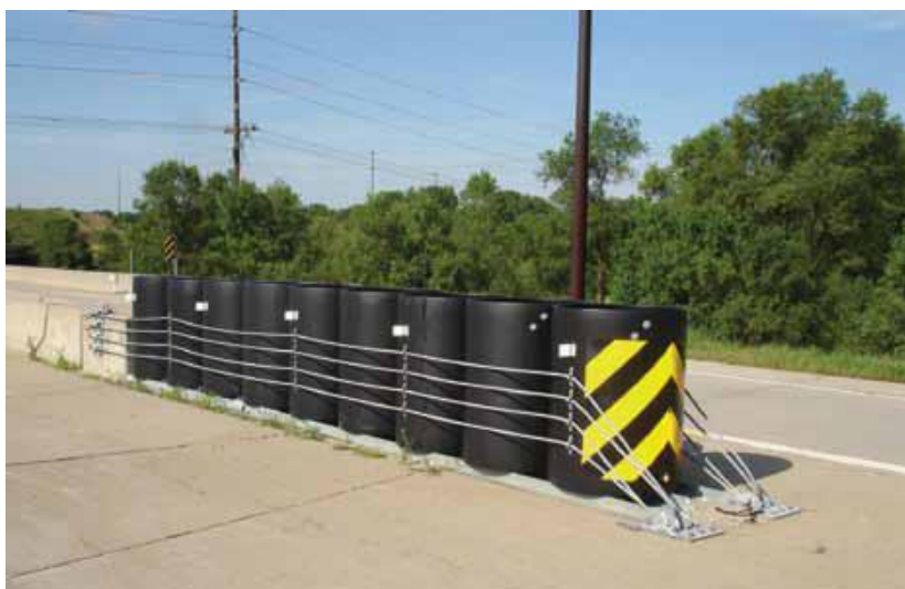
Plate 12.36 Reusable Energy-Absorbing Crash Terminal (REACT 350®)
