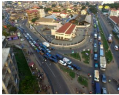
(b) Poor delineated slip lane
