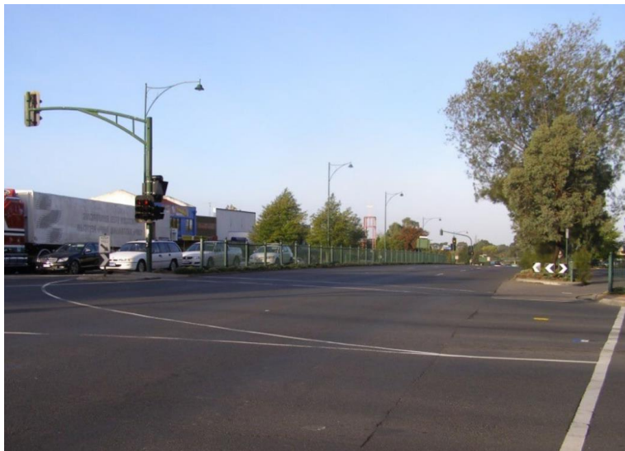
Plate 12.40 Median fence directing pedestrians to controlled crossings
