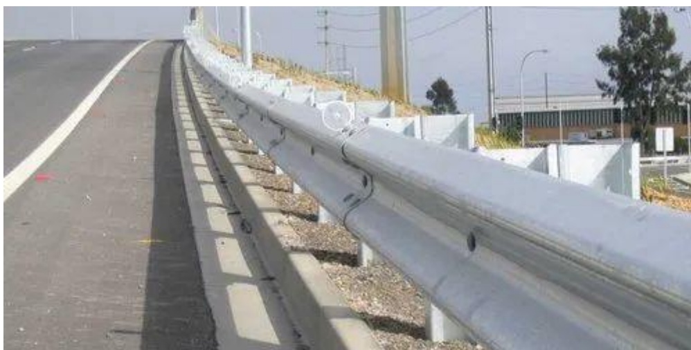
Plate 5.36 Rail units overlap in the wrong way
