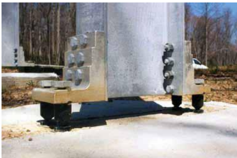
Plate 12.52 Multidirectional coupler
