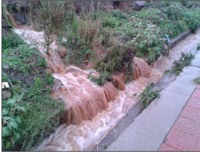
Plate 13.5 Roadside drain collecting lateral flows
