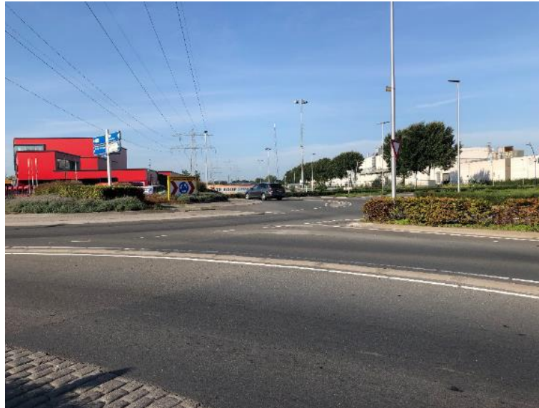
Plate 8.18 Raised lane divider in a turbo roundabout in the Netherlands.
