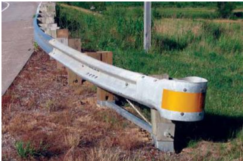
Plate 12.19 Modified eccentric loader terminal (MELT)
