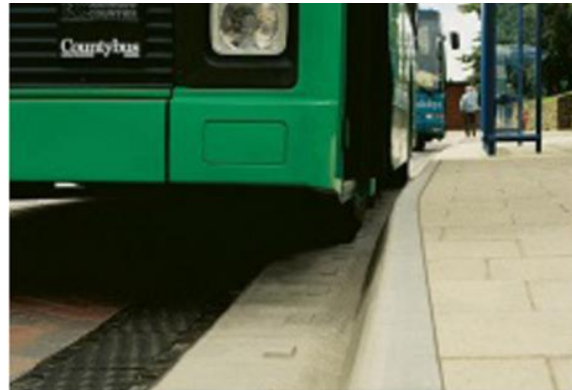
Plate 5.42 Non-mountable kerb adjacent to walkway and lay-by
