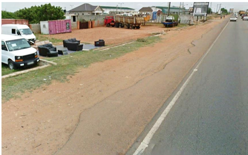
Plate 5.22 Pavement edge drop along the shoulder
