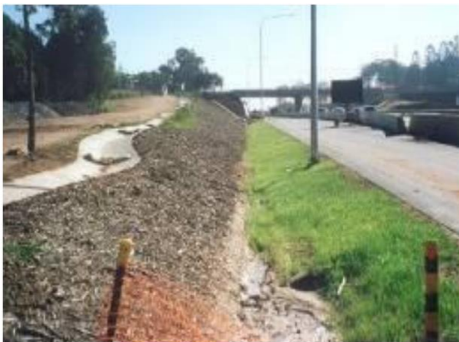
Plate 13.7 Concrete-lined catch drain
