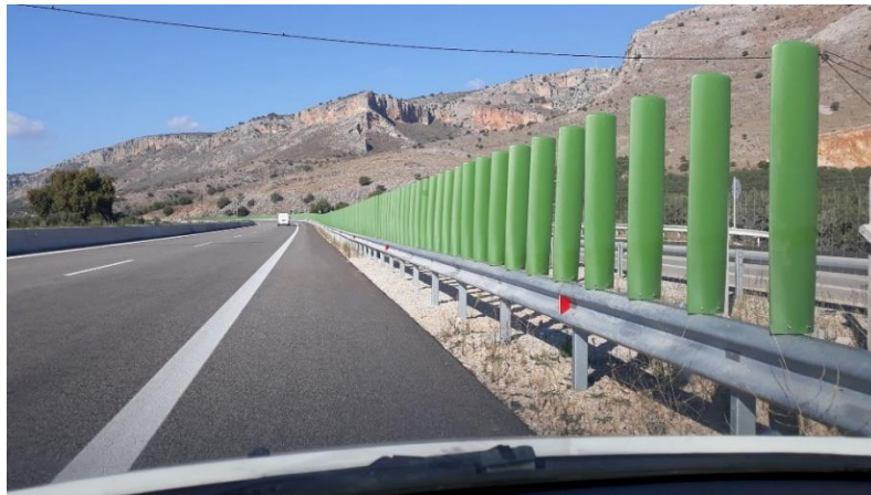
Plate 12.48 Safety barrier mounted Anti-Glare Screens
