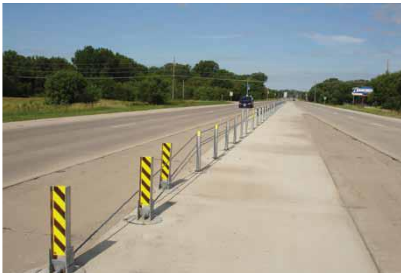
Plate 12.17 CASS TM cable terminal (CCT)
