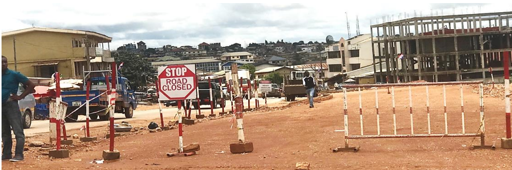
Plate 5.3 Poor barricade and sub-standard stop/“road closed” sign
