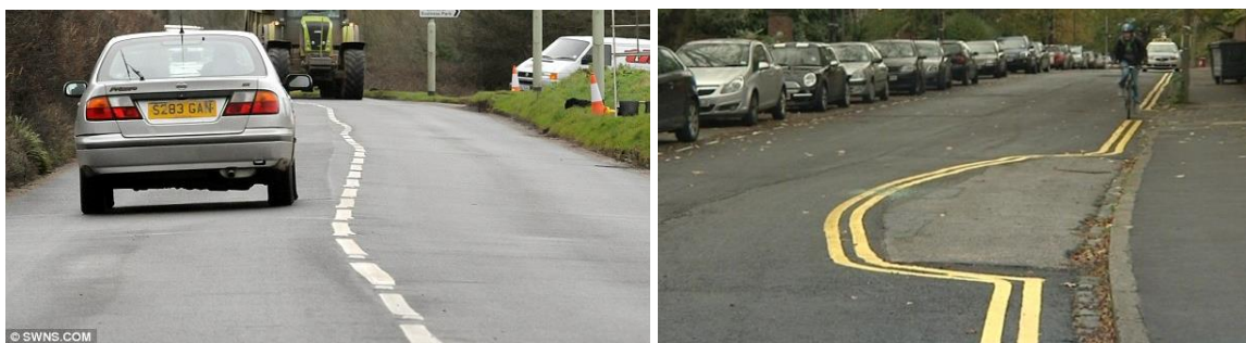
Plate 5.45 Unexpected deviation of line marking
