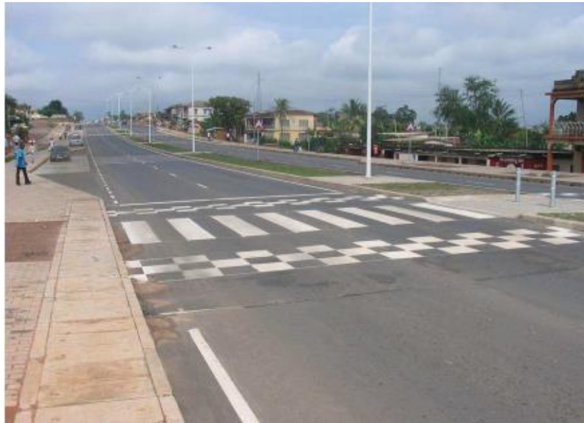
Plate 10.1 Trapezoidal hump in asphalt, near Kumasi.
